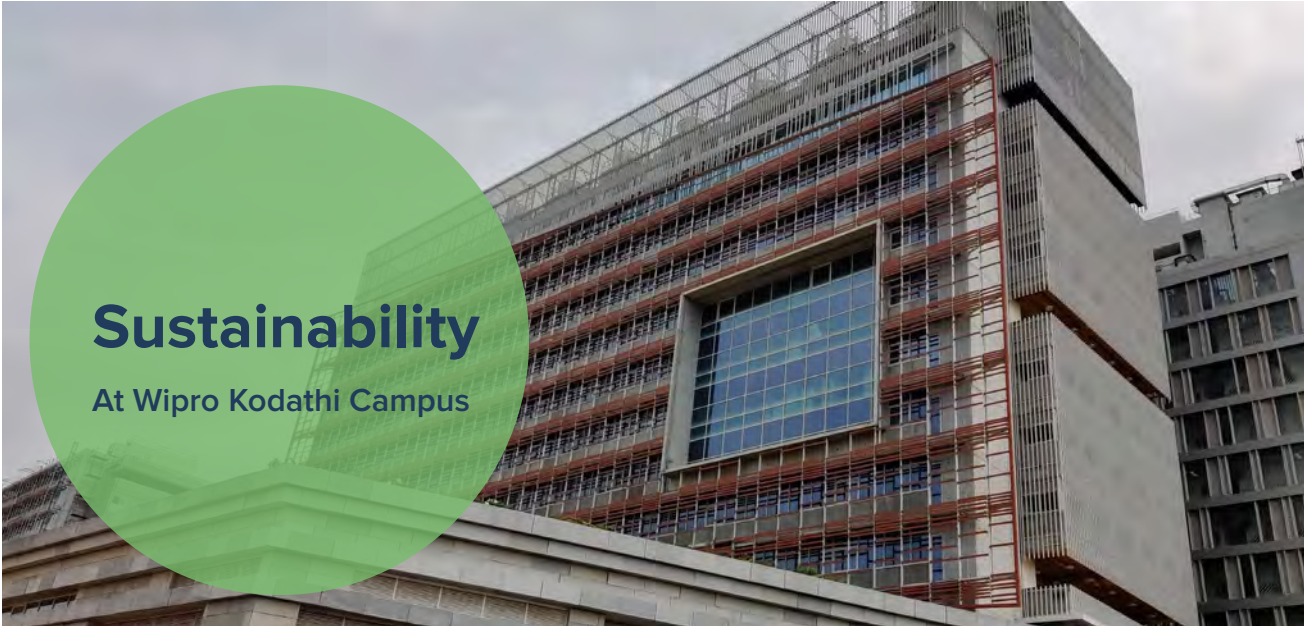
The building's design and orientation are based on the sun path, and it has a double-skinned façade to reduce heat ingress.
