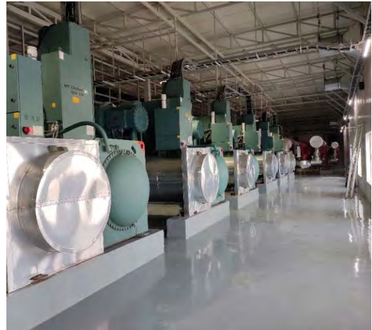
Energy efficient magnetic bearing centrifugal chillers
