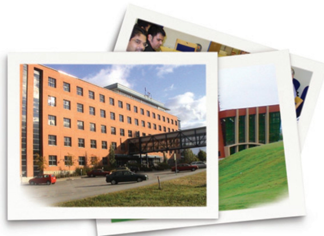
Wipro Development Center at Finland
