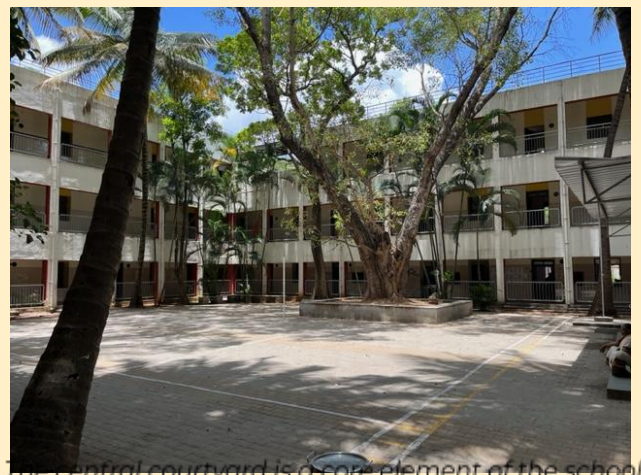
The central courtyard is a core element of the school
