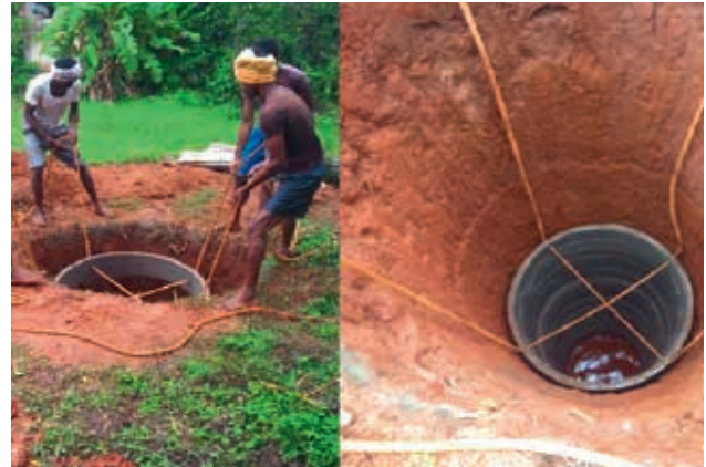
A new open well in the community
