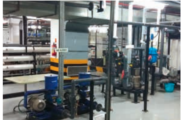
Ultra filtration unit at one of our locations
